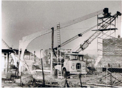
Construction work well under way
