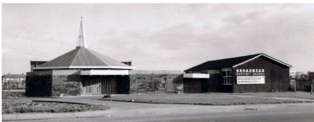
The new church building on completion
